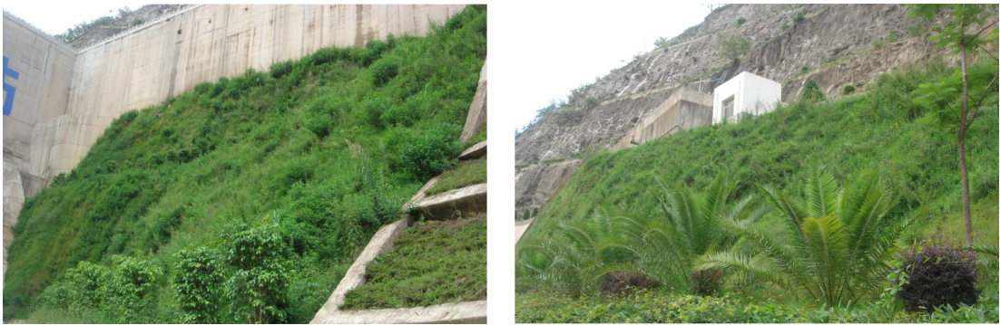
图 3 生物防护边坡的整体效果 Fig.3 The overall effect of biological protection of slope
