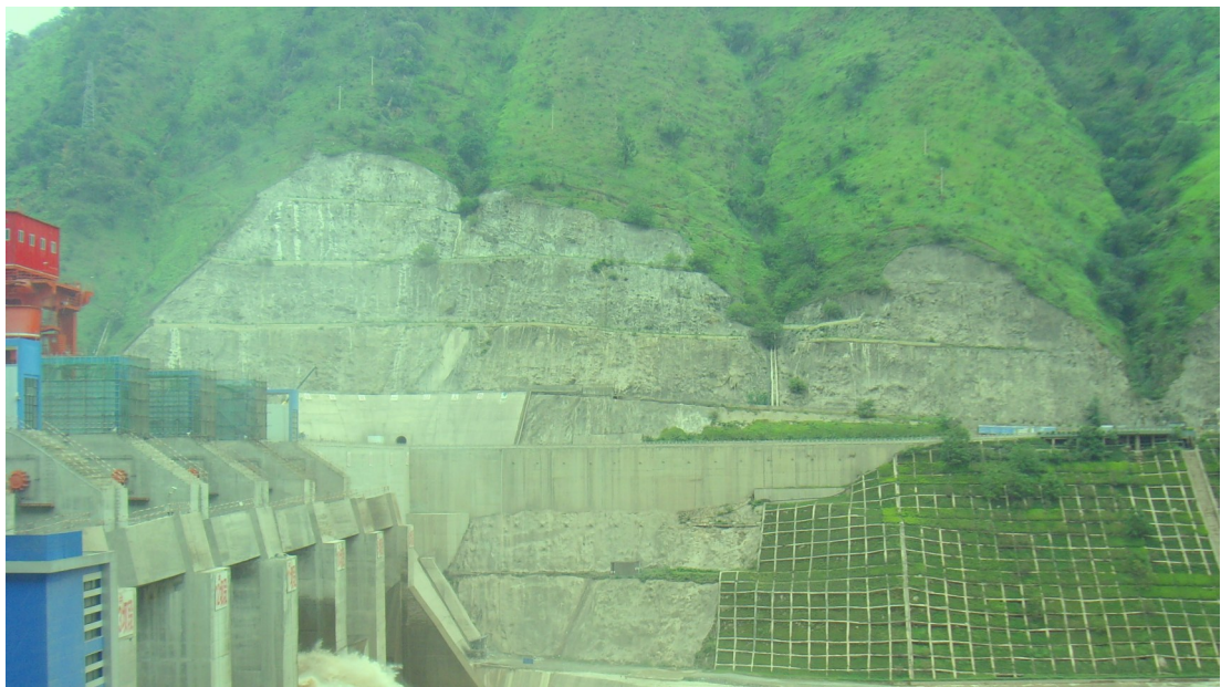
图 2 观礼台上边坡及坝后左岸边坡 Fig.2 The reviewing stand behind the dam slope and the slope on the left bank
